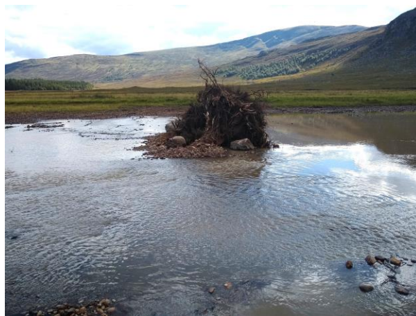
A few weeks after installation
