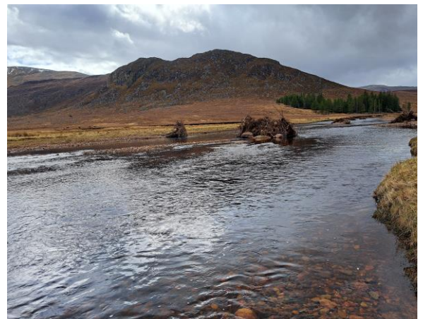
7 months after installation showing gravel deposition downstream of LWS
